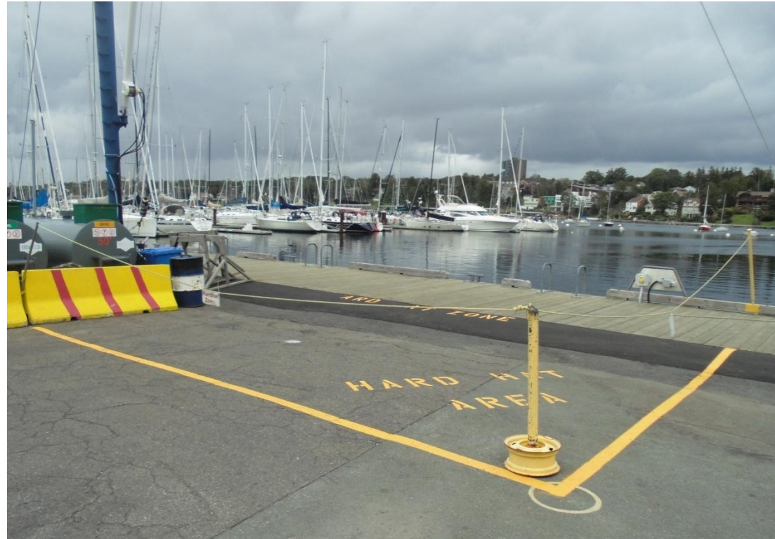
Spar Crane Safety line demarcation
